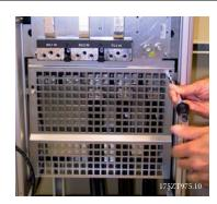
Figure 3.52: Mount the EMC shield.
