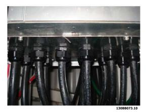
Figure 3.32: Example of proper installation of the connector plate.
